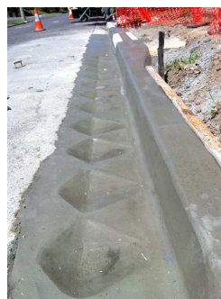
Sediment grooves during construction
