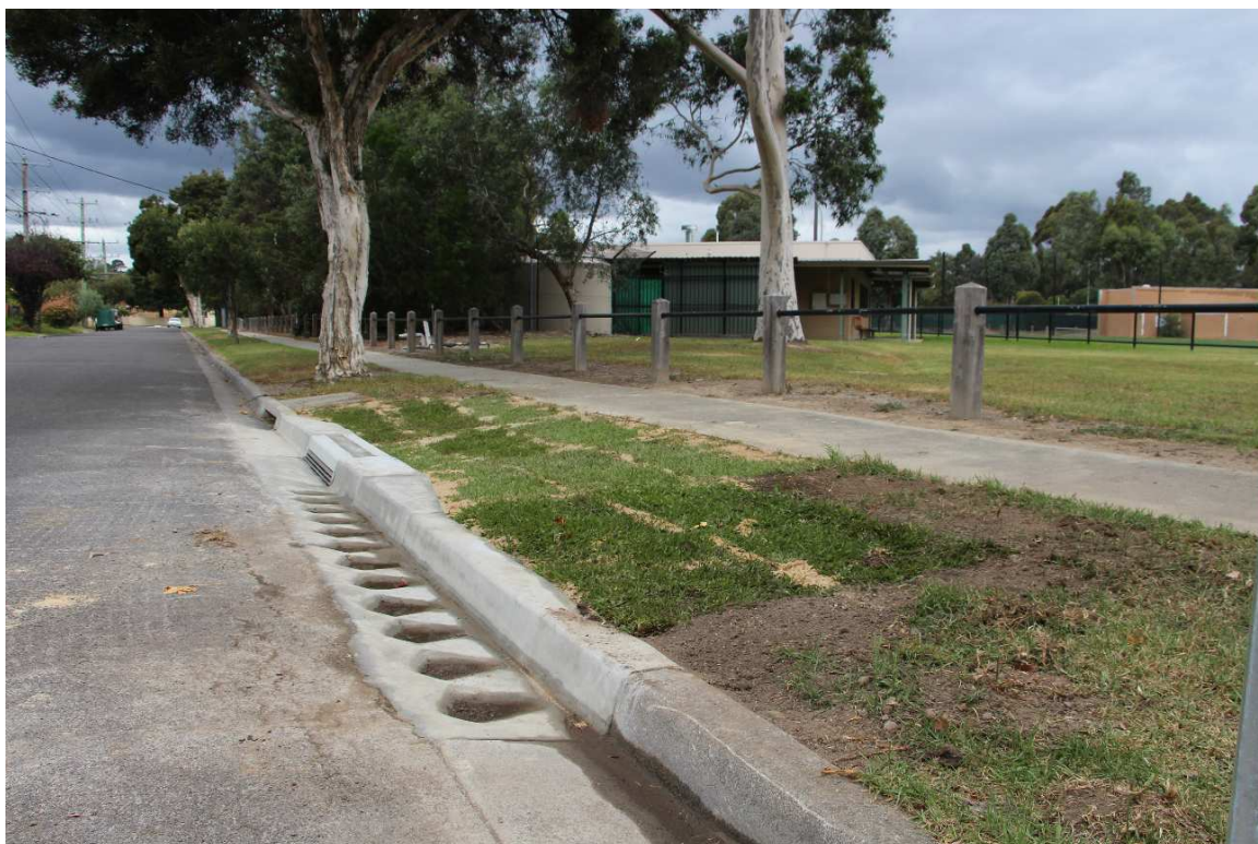
Park Avenue, Doncaster, single barrier kerb installation
