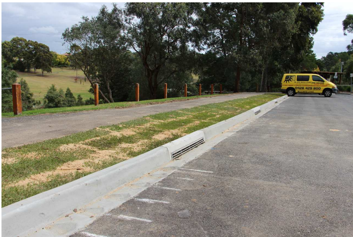
Ruffey Lake Park, Victoria Street car park, Doncaster, barrier kerb installations (5 no.)
