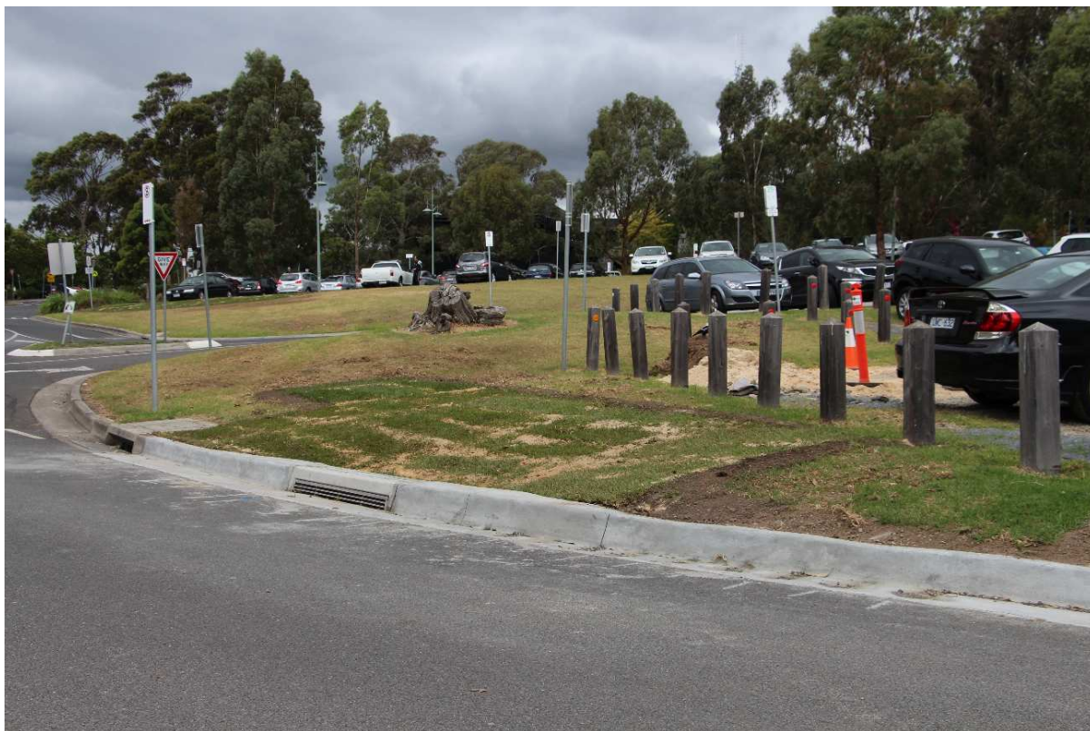
Hummel Way, Doncaster, single barrier kerb installation
