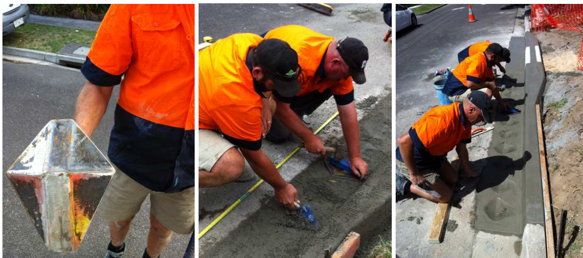
Sediment groove installation, Park Avenue, Doncaster
