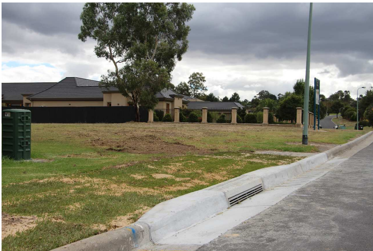
Edwin Street, Templestowe, single barrier kerb installation
